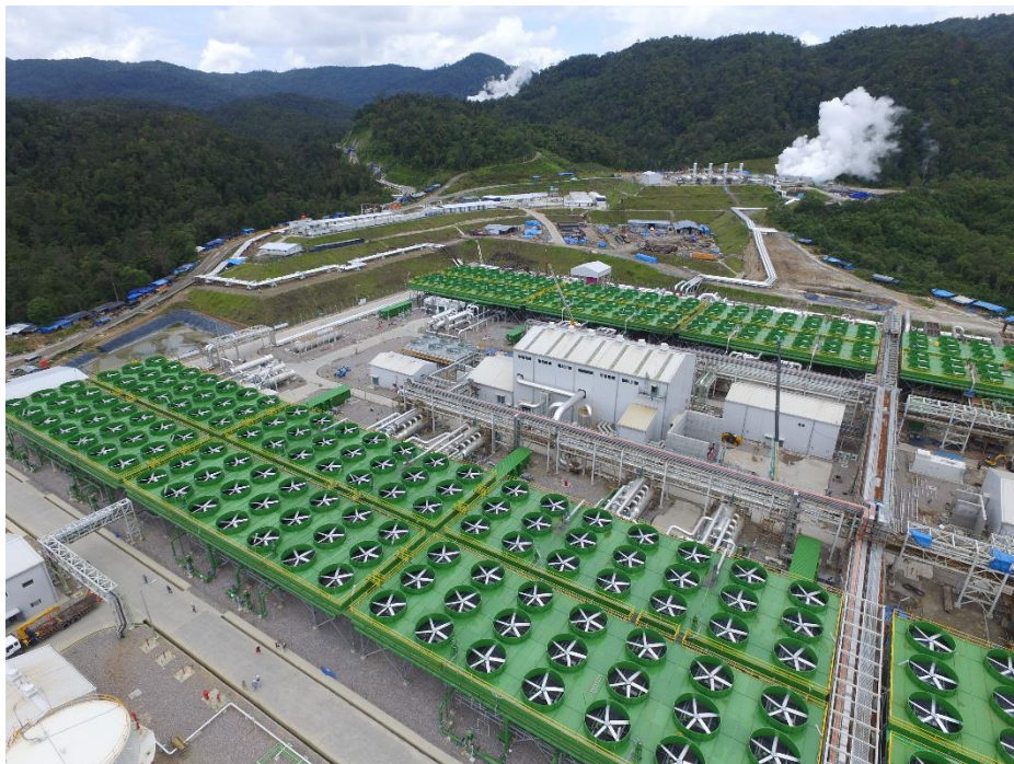
The second unit of Sarulla Geothermal IPP project
