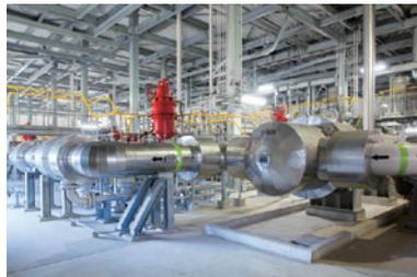
This facility adjusts the calorific value of regasified LNG and natural gas produced in Japan by adding liquefied petroleum gas (LPG). The end product is then transferred to the pipeline network as sales gas.
