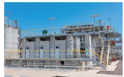
ORH uses seawater as heat source to heat the cryogenic LPG at  $-43^{\circ}\text{C}$  to ambient temperature.
