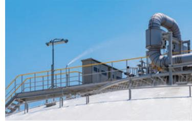
A sprinkler system is installed on LNG, cryogenic LPG and ambient LPG tanks. In the event of a fire, the system will spray water to cool the tanks protecting them from the radiant heat. The equipment will also prevent the fire from deforming structures and spreading to adjacent facilities.
