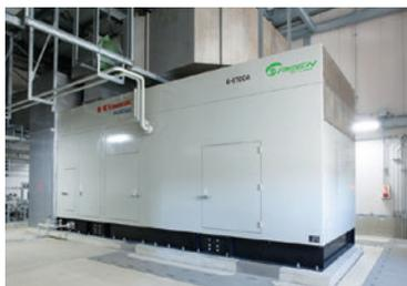
The terminal has generators to cope with power outages. The diesel generator is a backup source of power to keep the terminal safe. If a power outage persists, the gas turbine generator is activated to sustain terminal operations.
