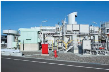
The SMV is a vaporizer operated mainly in emergencies. It burns natural gas to create high-temperature exhaust gas that heats water in a tank containing heated tubes that regasify the LNG through heat conduction.
