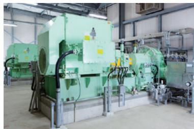
RGB is used to transfer boil off gas (BOG) to unloading LNG vessels to maintain positive pressure inside the cargo tank.
