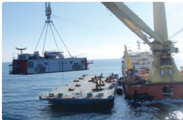
Removing above-water structures of the platform
