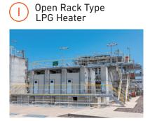
ORH uses seawater as heat source to heat the cryogenic LPG at -43 °C to ambient temperature.
