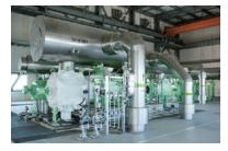
Boil off gas (BOG) is constantly produced in the LNG and cryogenic LPG tanks due to heat flux from the surroundings. There are two ways to process the LNG BOG. One is to re-liquefy the gas and transfer it back to the tank or vaporizer. The other is to compress the BOG and send it to a vaporized gas pipeline. LPG BOG is processed by re-liquefying it and sending it to either the ambient temperature LPG tank or cryogenic LPG tank.
