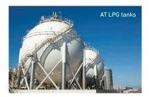
LPG is used in calorific adjustment. There are two types of LPG storage tanks; ambient temperature LPG tank and cryogenic LPG tank.
