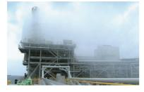
In the event of a fire during unloading operations, a water curtain over 20min height is deployed to prevent radiant heat from affecting vessels and adjacent facilities at the terminal. Vaporized gas will also be diffused upward to quickly lower the density of gas at ground level.
