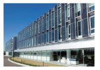
High-efficiency polycrystalline solar panels are installed on the south-east walls and roofs of the administration building and pipeline operations center. The panels which also function in snowy conditions, produce electricity that partially powers the buildings.
