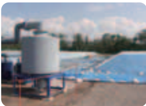
Biopile remediation for soil decontamination
