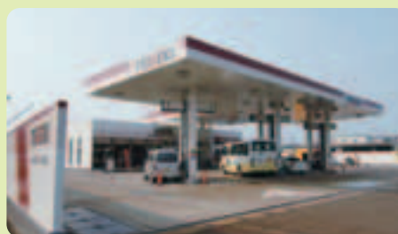
Service station in Oogata
