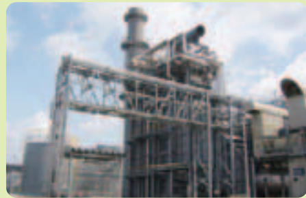
Koshijihara Power Plant
