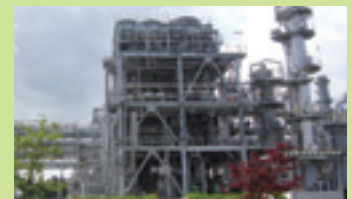
Gas-processing facility at the Koshijihara Plant
