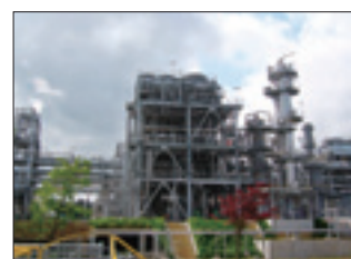
New processing train at a gas plant
