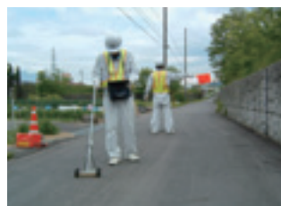
Leakage detection with FID gas detector
