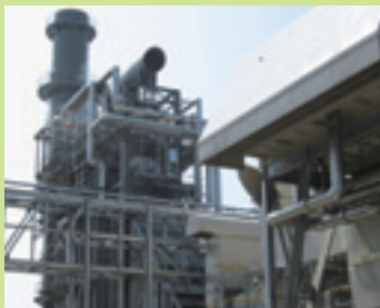
The Koshijihara Power Plant
