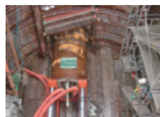
Construction of gas pipeline
