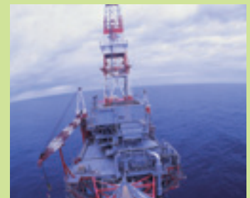
Platform at the Offshore Iwaki Gas Field
