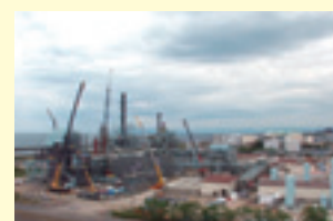
GTL demonstration plant under construction
