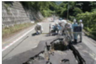
Inspecting damages to a road under which pipelines run
