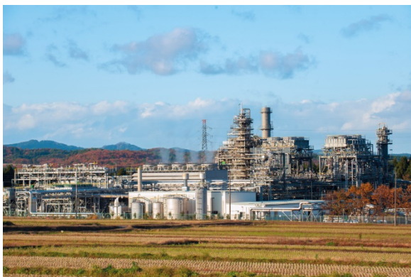
Koshijihara Plant at the Nagaoka Field
