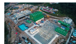
Muara Laboh Geothermal Power Plant
