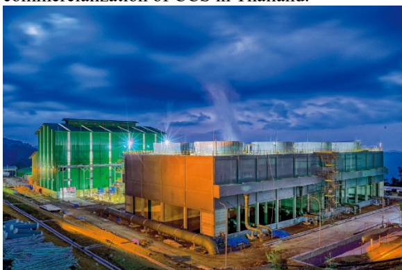
Muara Laboh Geothermal Power Plant
