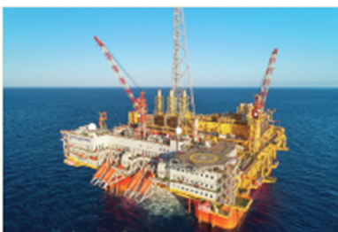
Offshore production and central processing facility (CPF)
