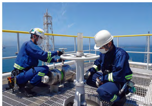
Wearing face shields and masks while working (Naoetsu LNG Terminal)
