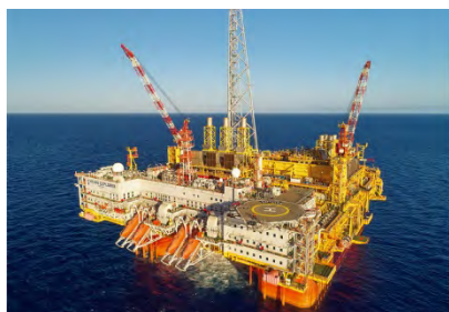
Offshore production and processing facility (CPF)
