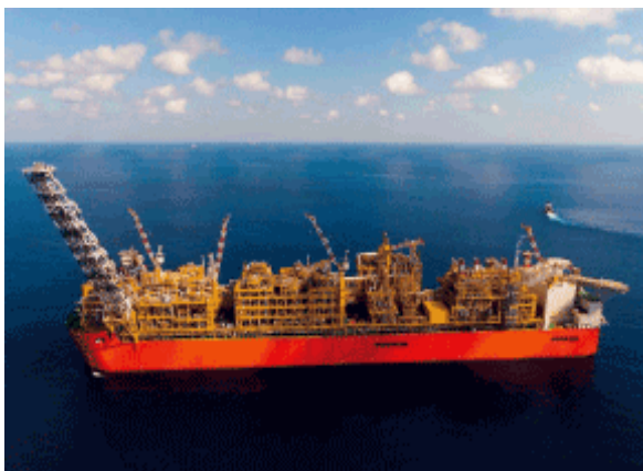
The Prelude FLNG facility
