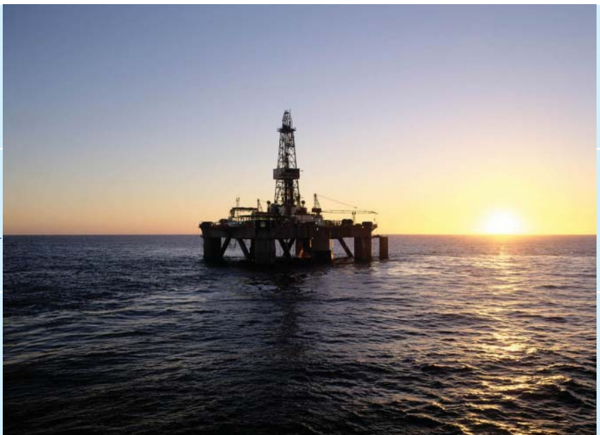
Drilling Rig, Timor Sea
