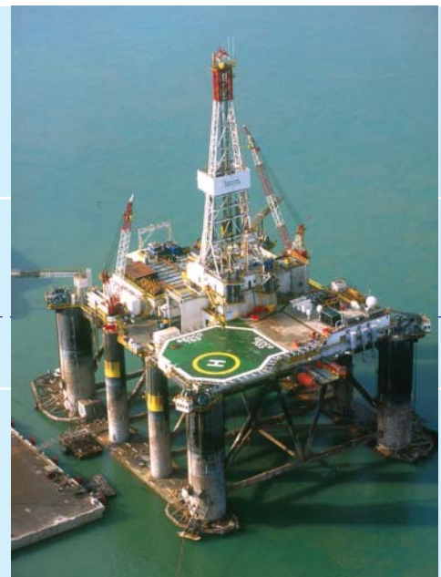
Drilling Rig, WA-285-P
