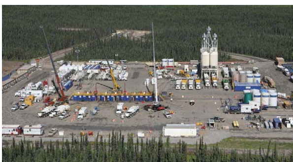
Hydraulic Fracturing site in the Horn River Area
