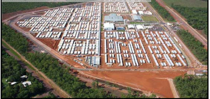
Accommodation Village in onshore LNG plant(Jan. 2014, in Darwin)
