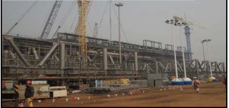
Fabrication of module for onshore LNG plant (Jan. 2014 in China)
