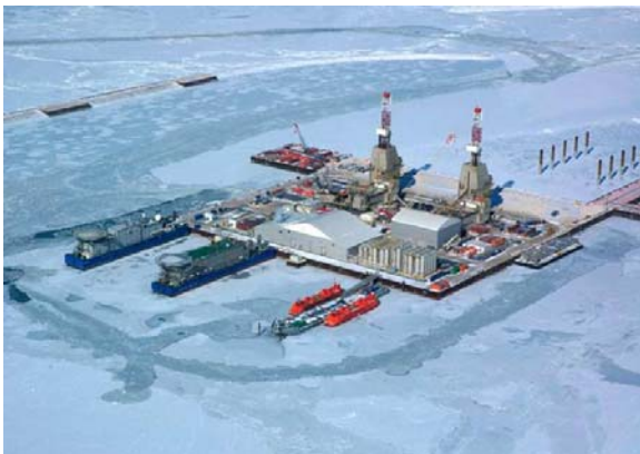
Offshore Production Facilities (Kashagan Oil Field)
