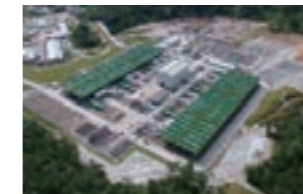
Sarulla Geothermal Independent Power Producer (IPP*) Project
