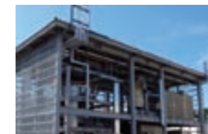
Testing facilities at the Koshijihara Plant (Niigata) (a NEDO project)
