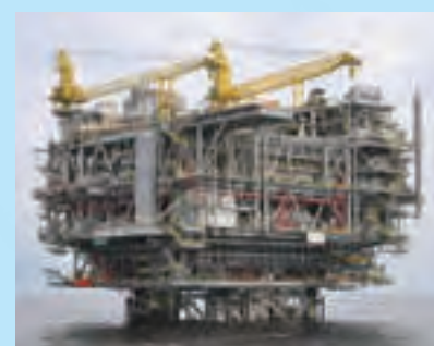
Offshore production facilities
