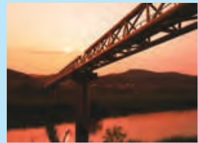
Natural gas pipeline crossing a river (Shibumi River, Niigata Prefecture)
