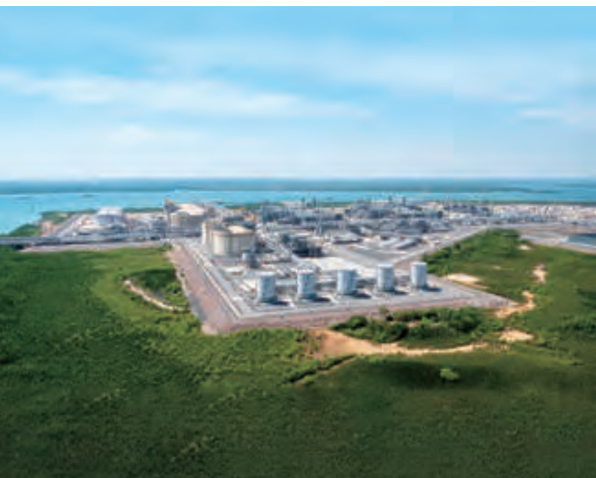
Ichthys LNG Project Onshore liquefaction plant in Darwin
