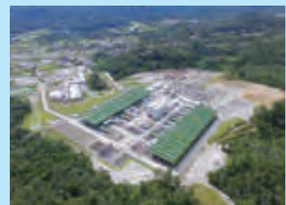
Sarulla Geothermal IPP Project
