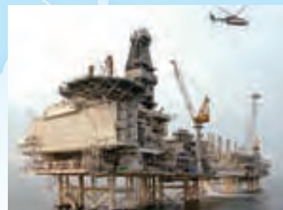
Offshore production facilities
