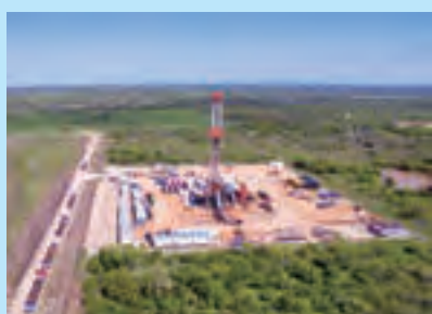
Drilling operations site
