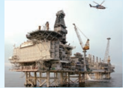
Offshore production facility
