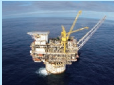
Offshore production facility in the Lucius Oil Field
