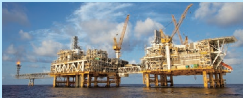
Bayu-Undan offshore facility
