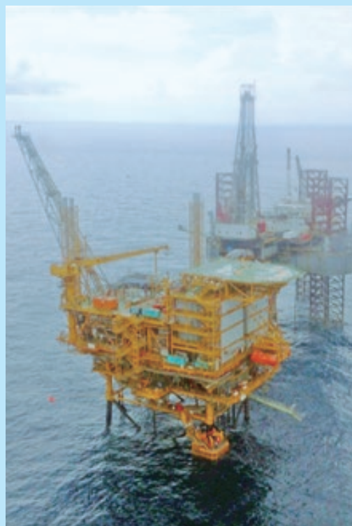
Offshore production facility in the Ruby Gas Field
