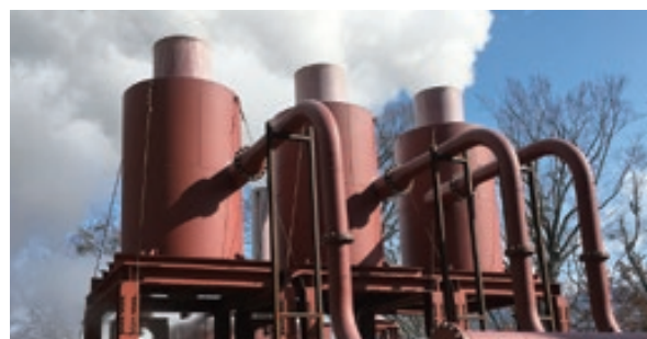
Geothermal flow tests in the Oyasu region in Akita Prefecture, Japan
