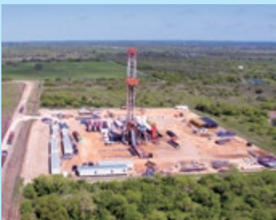
Drilling operations site
