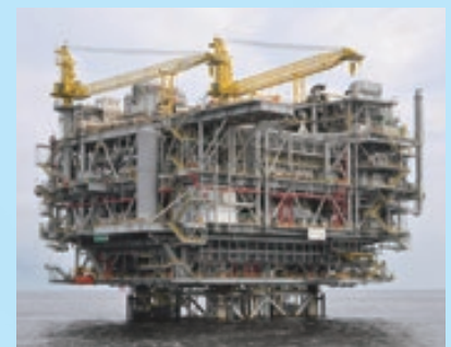
Offshore production facility
