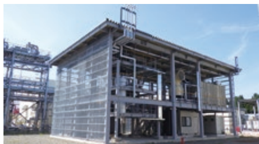
CO 2 methanation test facility currently under construction
