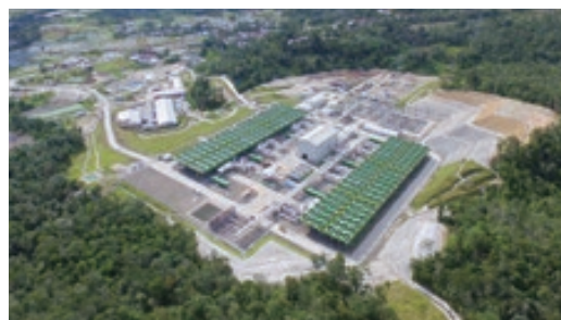
Indonesia Sarulla Geothermal IPP Project
