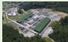
First unit of the Sarrula Geothermal IPP Project
