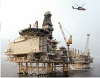
Offshore production facilities
