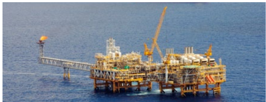
Bayu-Undan offshore facility
