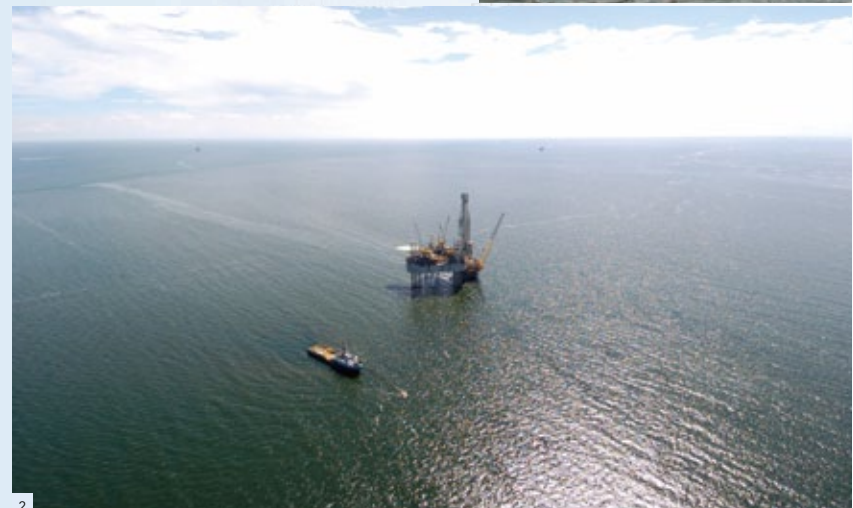
1: Booster station 2: Offshore platform during well drilling work
