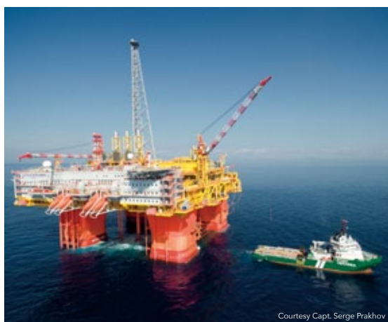
CPF (Ichthys Explorer) undergoing mooring operations
