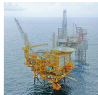
Offshore production facility in the Ruby Gas Field
