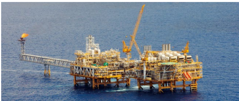
Bayu-Undan offshore facility
