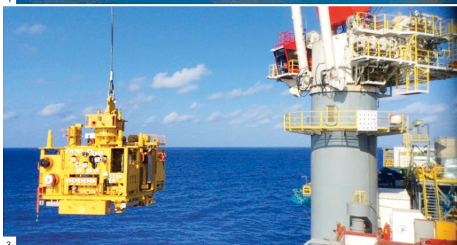
1: FPSO under construction 2: ENSCO5006 drilling rig for a production well 3: Subsea wellhead assembly installation operations 4: CPF under construction
