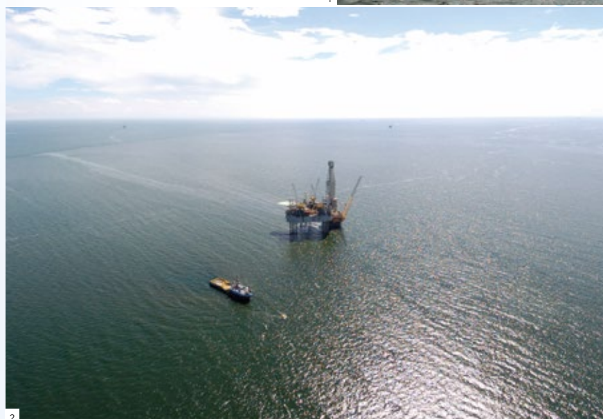
1: Compression unit 2: Production facility
