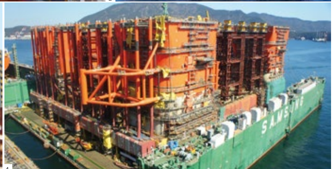
1: FPSO under construction 2: ENSCO5006 drilling rig for a production well 3: Subsea wellhead assembly 4: CPF construction at floating dock
