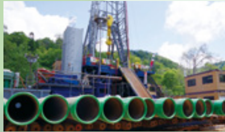
Exploratory well drilling work for geothermal energy development in the Amematsudake region (July 2013)
