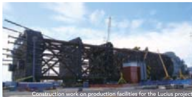
Construction work on production facilities for the Lucius project
