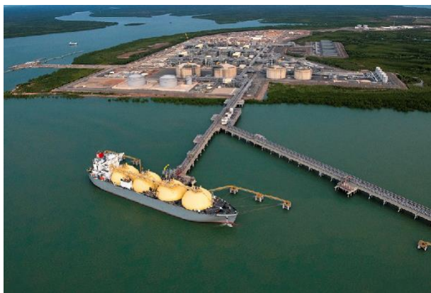
Ichthys onshore production plant
