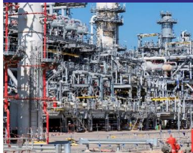
Ichthys onshore gas liquefaction plant
