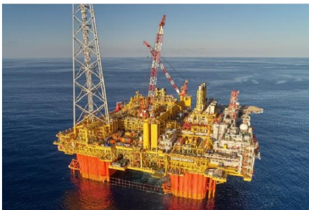
Central Processing Facility (offshore Australia)
