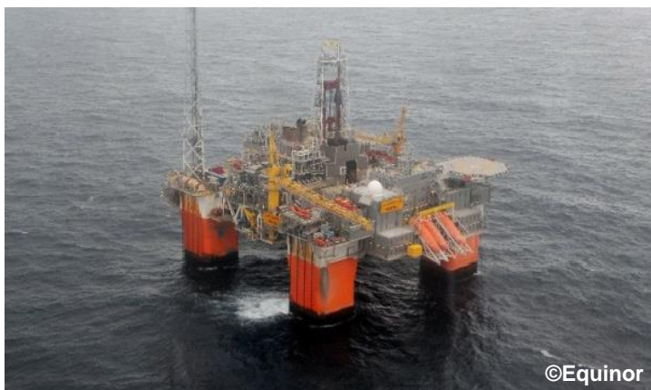
Offshore production facilities (Snorre Project)
