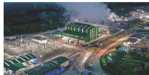
Muara Laboh Geothermal Power Project
