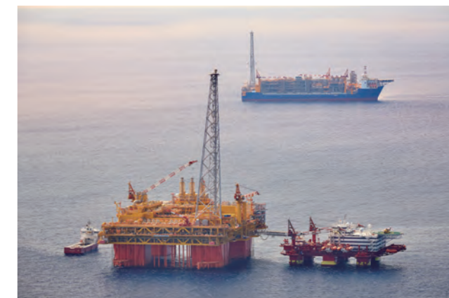
CPF and FPSO onsite
