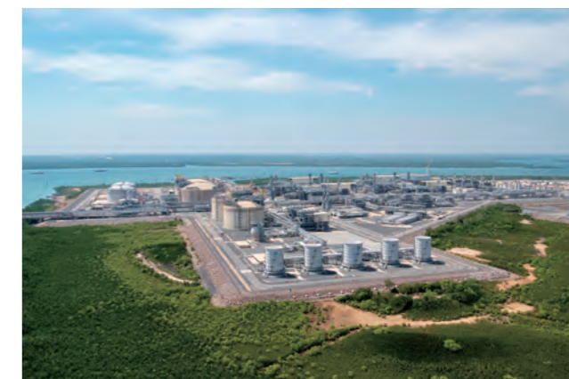
Panoramic view of onshore LNG plant
