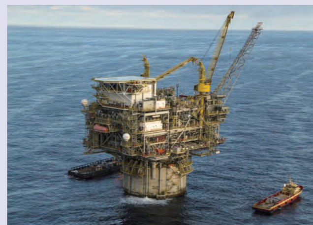
Production facilities at the Lucius Oil Field
