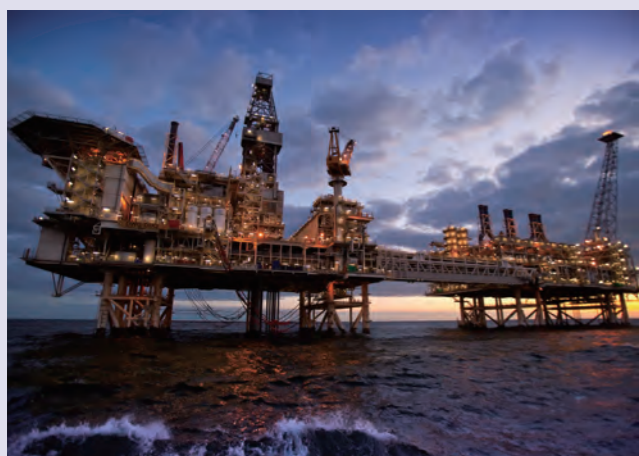
Production facilities at the ACG oil field concession in the Caspian Sea
