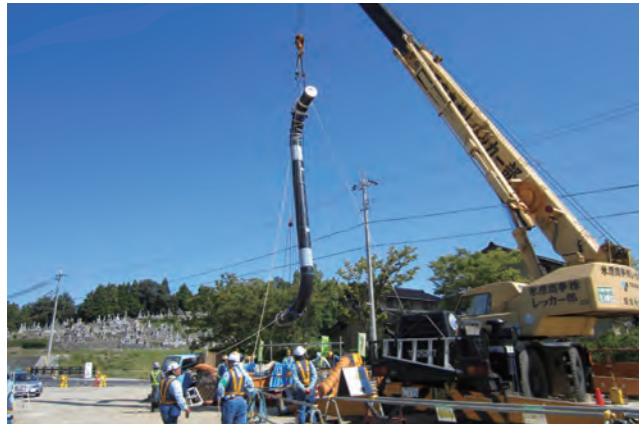
Toyama Line construction
