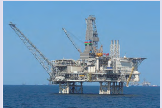
Production platform for the Chirag Oil Project in the ACG oil fields concession in the Caspian Sea
