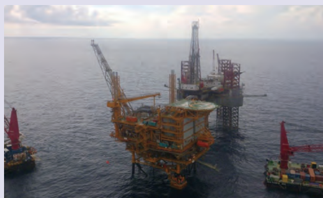
Oil production started in the offshore production facilities at the Ruby Gas Field, Indonesia
