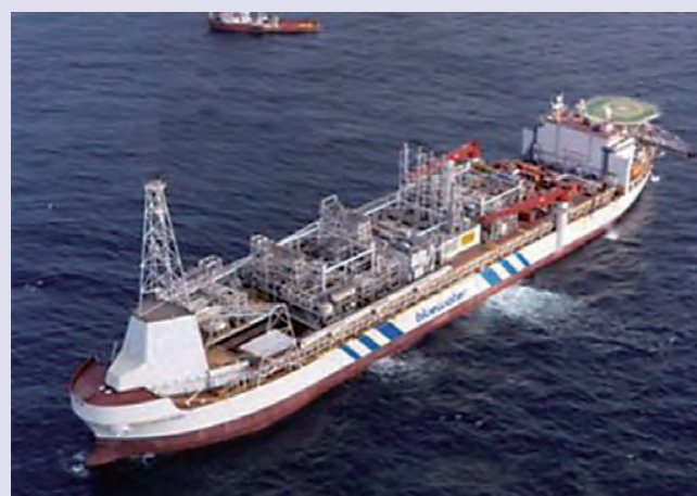
Oil production started at the Kitan Oil Field
