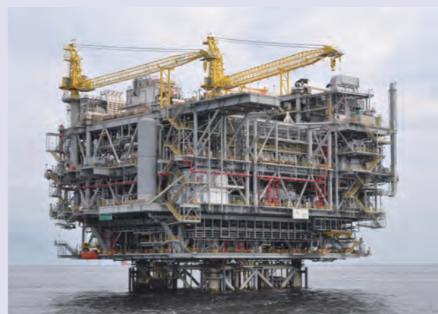
Production facilities at the Offshore Angola Block 14
